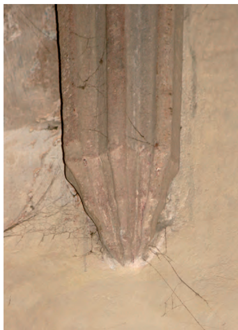
Obr. 17 Ostruhová konzola klenby v kostele sv. Václava v Moravské Ostravě, foto, 2010 Fig. 17 Spur shaped vault-console, St. Venceslaus church in Moravian Ostrava (part of Ostrava city), photo, 2010
